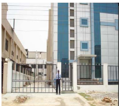
Front View of Warehouse
